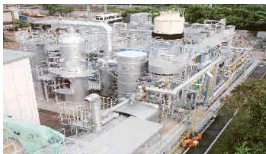
Figure 12 - Gasified MSW Fueled PAFC Power Plant
