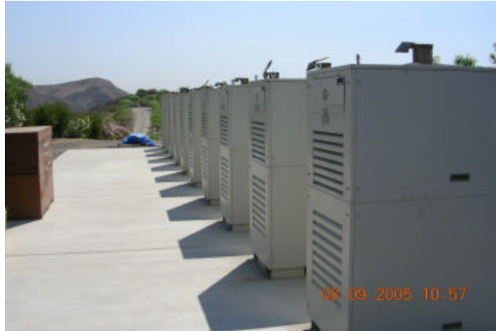
Figure 4. Microturbine Enclosures
